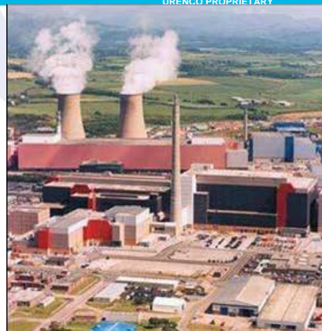
BNFL Thorp Reprocessing Plant in Sellafield United Kingdom
