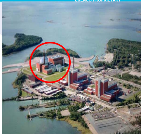
EPR Olkiluoto-3 (1600 MWe) Finland
