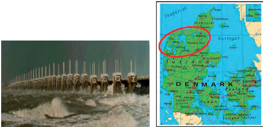
Figure 8.5. (left) The spring tide barrier. Figure 8.6. (right) Limfjorden Area (Denmark).
